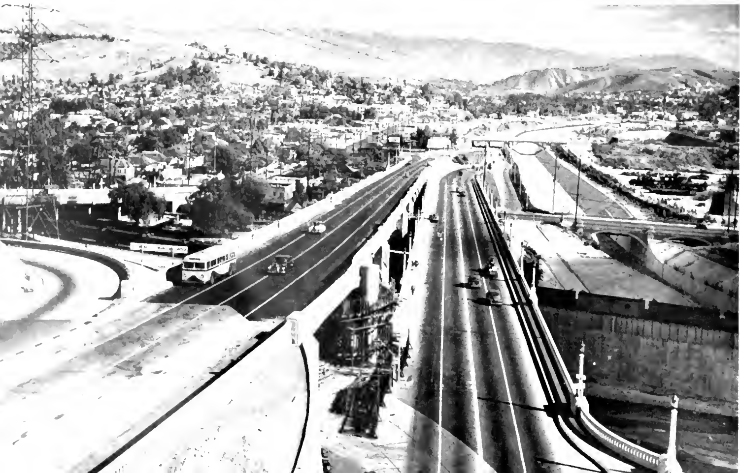
The newly completed Arroyo Seco Parkway Extension viaduct and bridge for southbound traffic only are shown at left of picture. Old viaduct and bridge over Los Angeles River for northbound traffic are seen at right.
